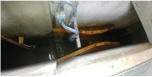
Figure 16: Headworks Building Influent Flowmeter
