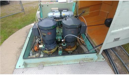
Figure 3: County Road Pump Station Pumps
