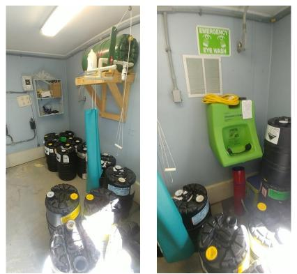
Figure 34 & 35: Disinfection Room Emergency Shower and Eye Wash Station
