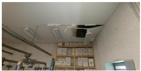
Figure 27: Blower Building Damaged Ceiling
