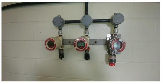
Figure 18: Headworks Building Gas Detection System
