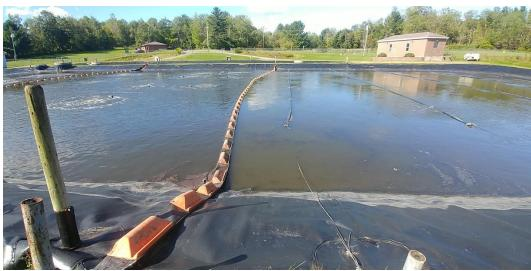
Figure 20: Lagoon #1 Baffle
